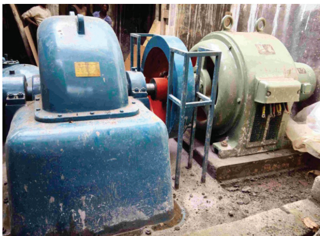
Kiliflora Project: Turbine and generator installation
