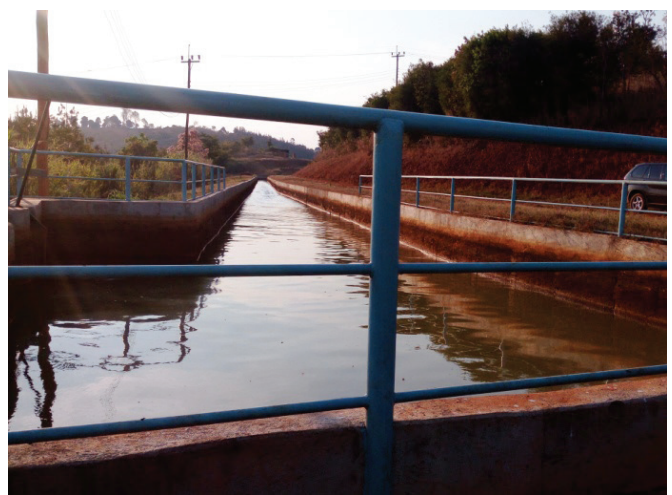
Andoya mini hydropower, Kifakara village, Mbinga District: Dam and headrace canal
