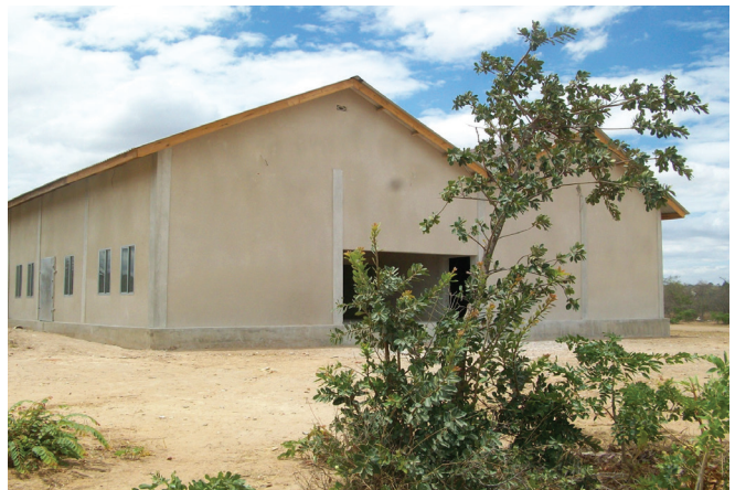
A modern abattoir being constructed by the Iringa Municipal Council
