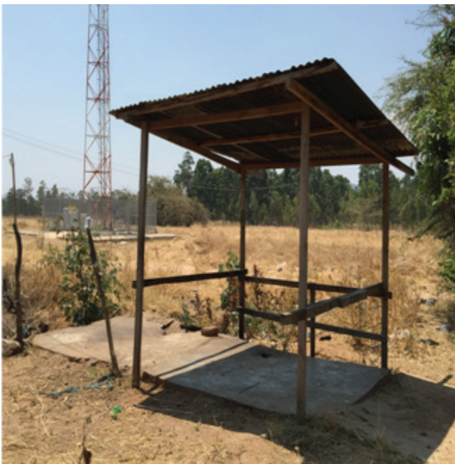
Slaughter shed at Nzihi village, Iringa District, before upgrading
