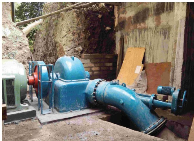
Kiliflora Project: Turbine and generator installation
