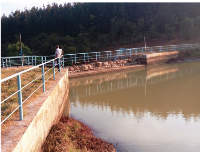
Andoya mini hydropower, Kifakara village, Mbinga District: Dam and headrace canal
