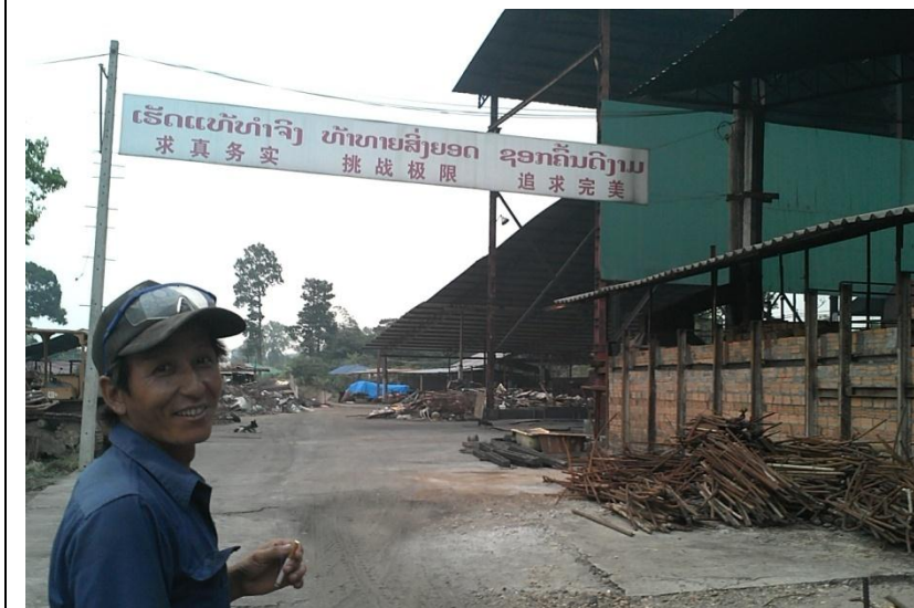
Saylong steel factory
