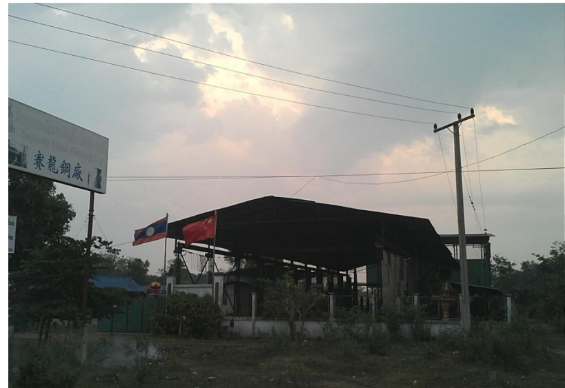
Saylong steel factory
