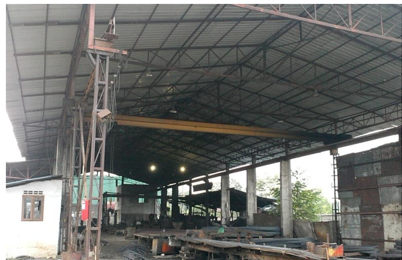
Saylong steel factory
