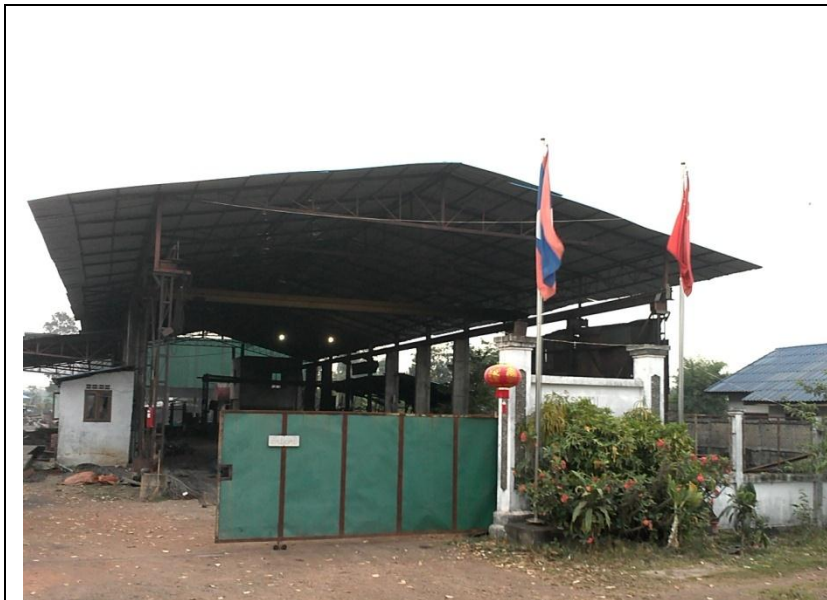
Saylong steel factory
