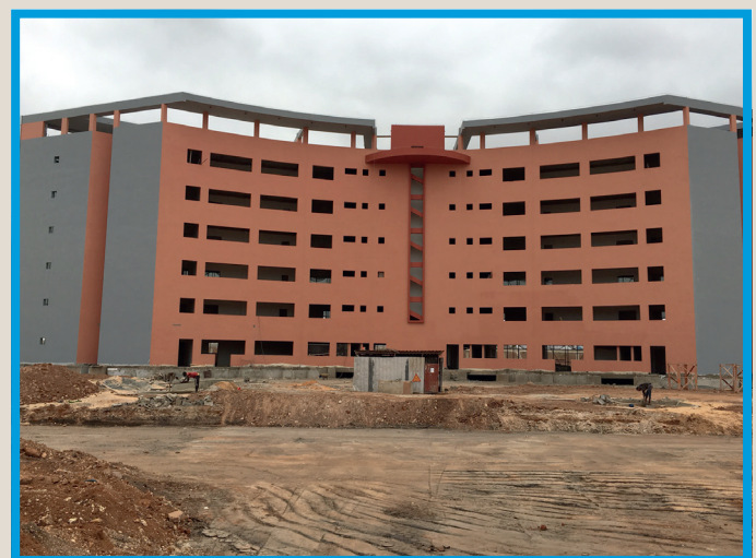
Figure 17: Commercial and administration building in Diamniadio Industrial Park, 12 July 2016
