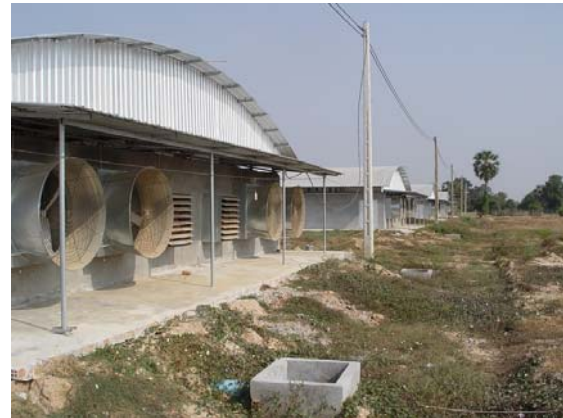
Figure 62: Fans in the back of a closed stable
