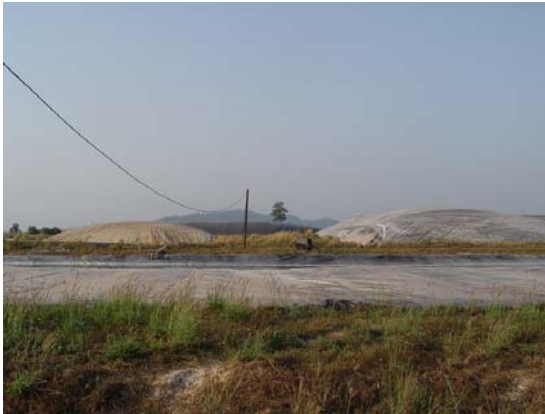
Figure 17: Covered lagoon digesters
