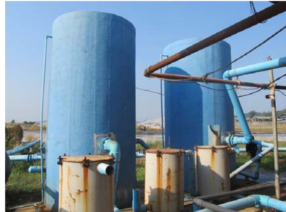
Figure 18: Gas treatment system
