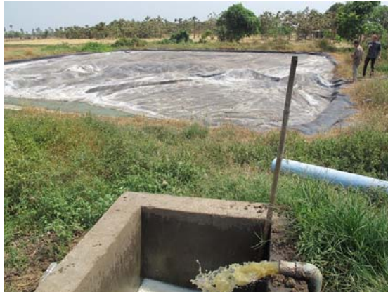
Figure 14: Sim Chanrith biogas plant
