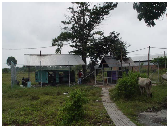
Figure 52: Generators at BVB
