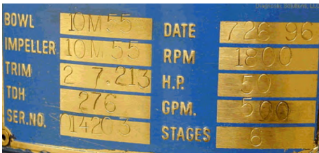
Fig. 12.1. Motor and Pump Nameplate Data
