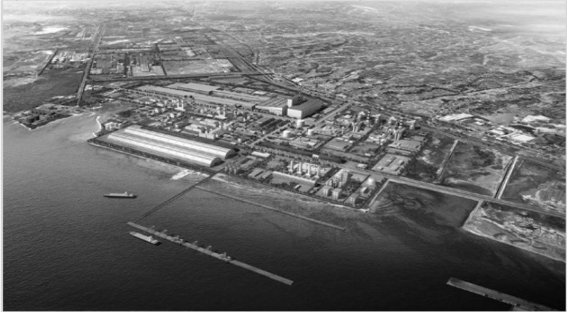
Figure 6-3-1. POSCO Steel Mill Bird's Eye View in Cilegon
