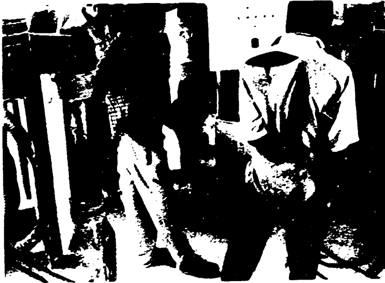
(26) JICA Expert is adjusting the distributor from 415V to 220V
