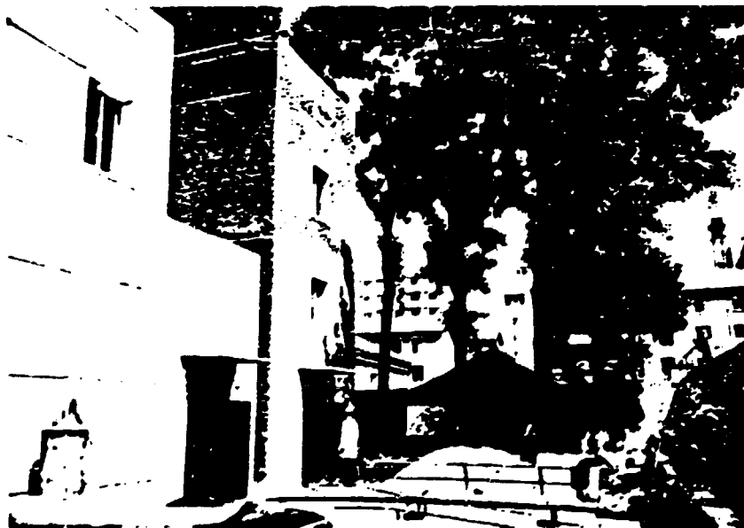
Fig. 2 General view of equipment hall and machine room in PEORC/Pyongyang
