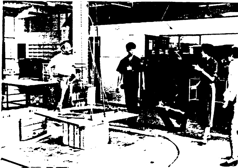
Compression tests of boxes size C40 and B100
