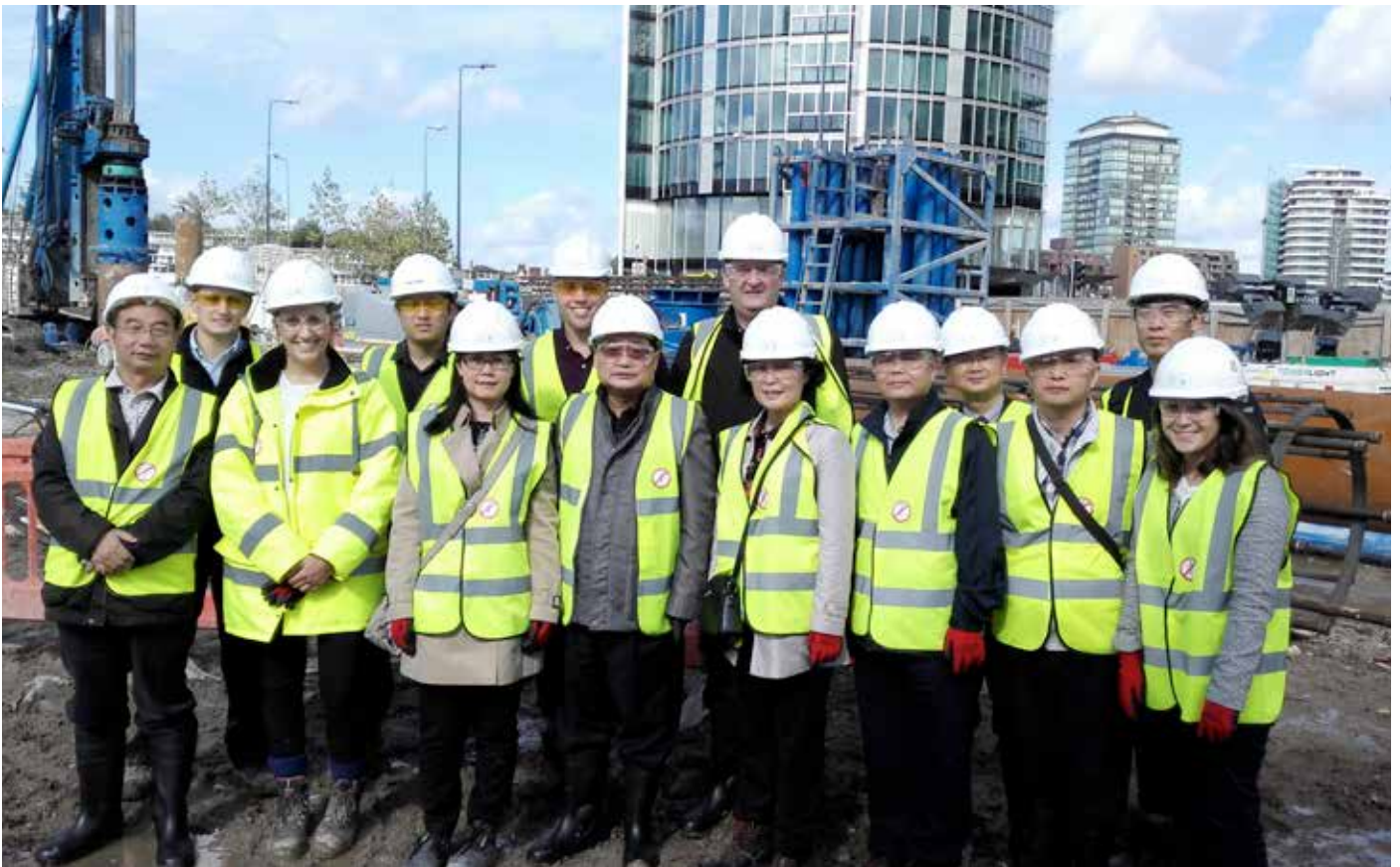
Participants of the study tour visit a construction site in London. LONDON, 2015
