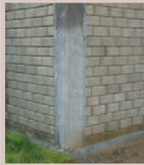
Joining together of horizontal reinforcement
