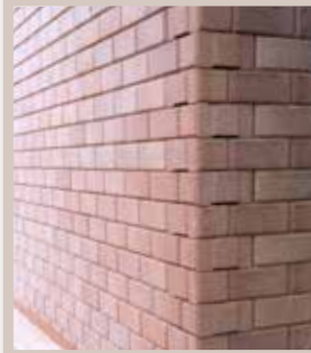
Use of half blocks at the corner of a wall
