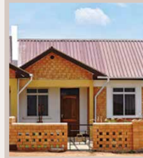
Residential house constructed from mud stabilized bricks/ blocks with a sloping roof
