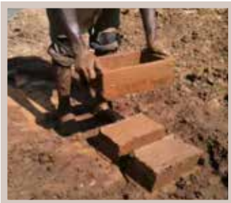
WOODEN MOULD FOR PRODUCING ADOBE BRICKS
