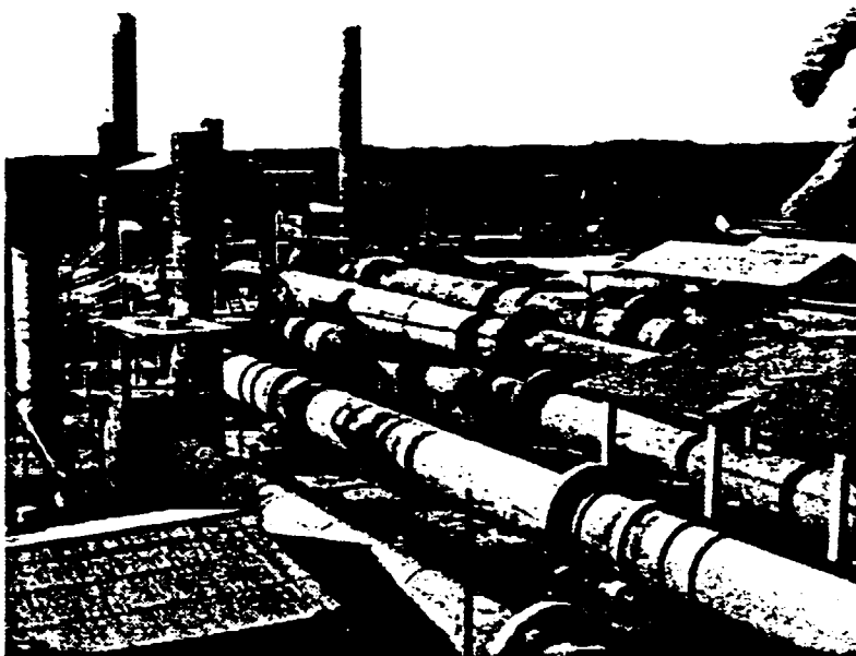
The five kilns of the plant - kiln no.1 in the foreground.
