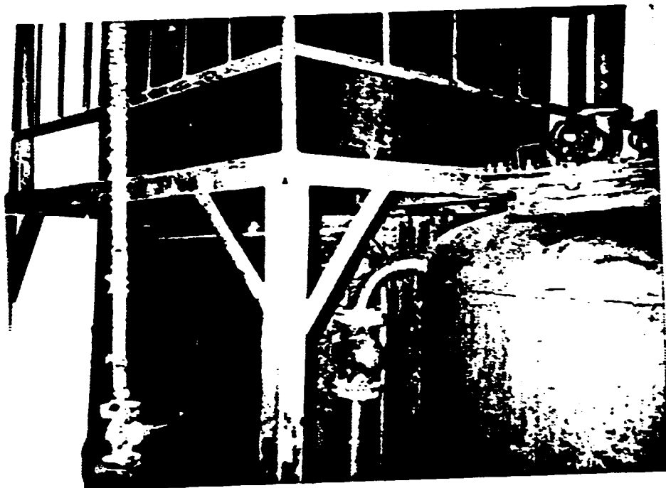
Rifampicin-Filtrate receiving tank
