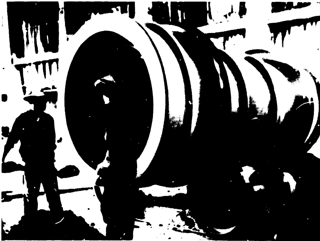
Figure 34. Pipe core feeding process
