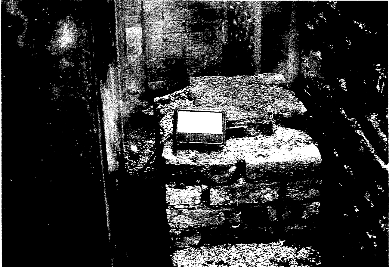
Figure 23. Pyrometer used to monitor the combustion process in the CRI incinerator
