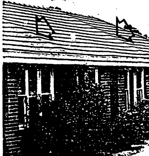
Figure 16 The whole appearance of these units has been spoilt because insufficient clearance was provided between the party walls and the roof system
