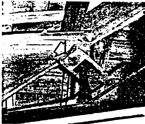
Figure 4 The steel prop goes part of the way towards making the Barap tie effective. Shrinkage of the packing piece, however, will tend to reduce the tie's effectiveness.
