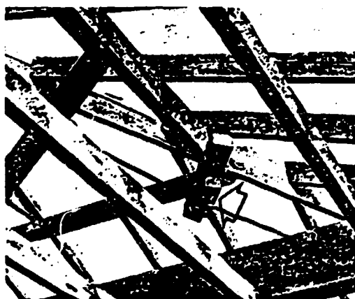
Figure 3 Green timber used on its edge as a prop for a Barap tie means that the tie becomes useless as the timber shrinks
