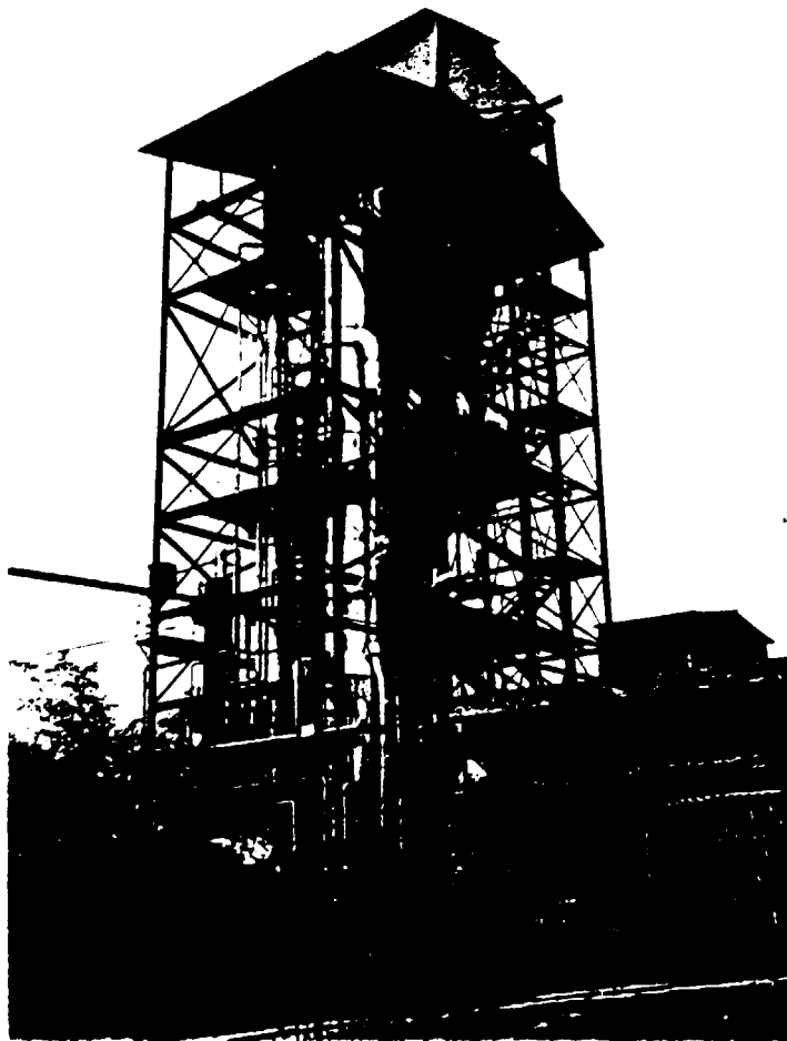
HOIST FOR COAL TRUCK TO GASIFIER BUNKER (top right)
