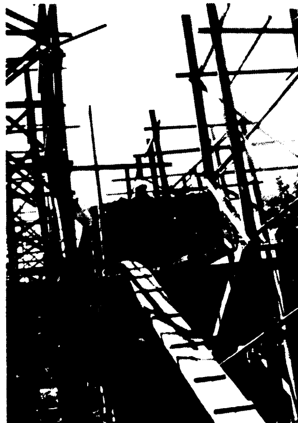
Figure 2 View of the scaffolding from the west side.
