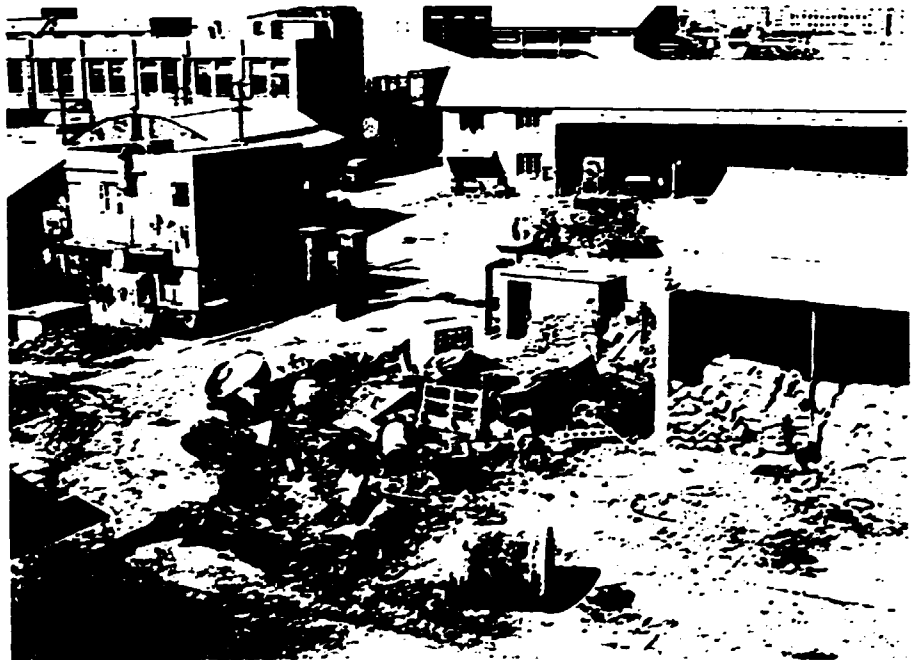
SCRAP DISMOUNTING AREA LABORATORY BUILDING
