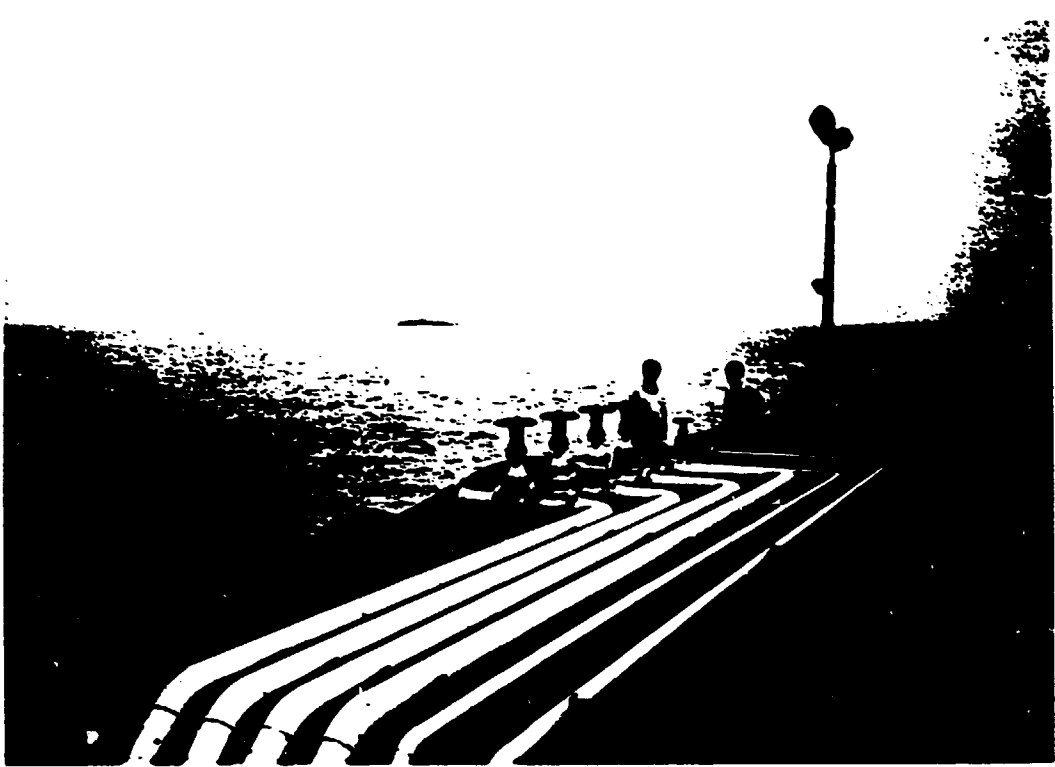
3. TANKER LOADING LINES - ONE FOR EACH PRODUCT PLUS A WATER LINE - NOT YET OPERATIONAL
