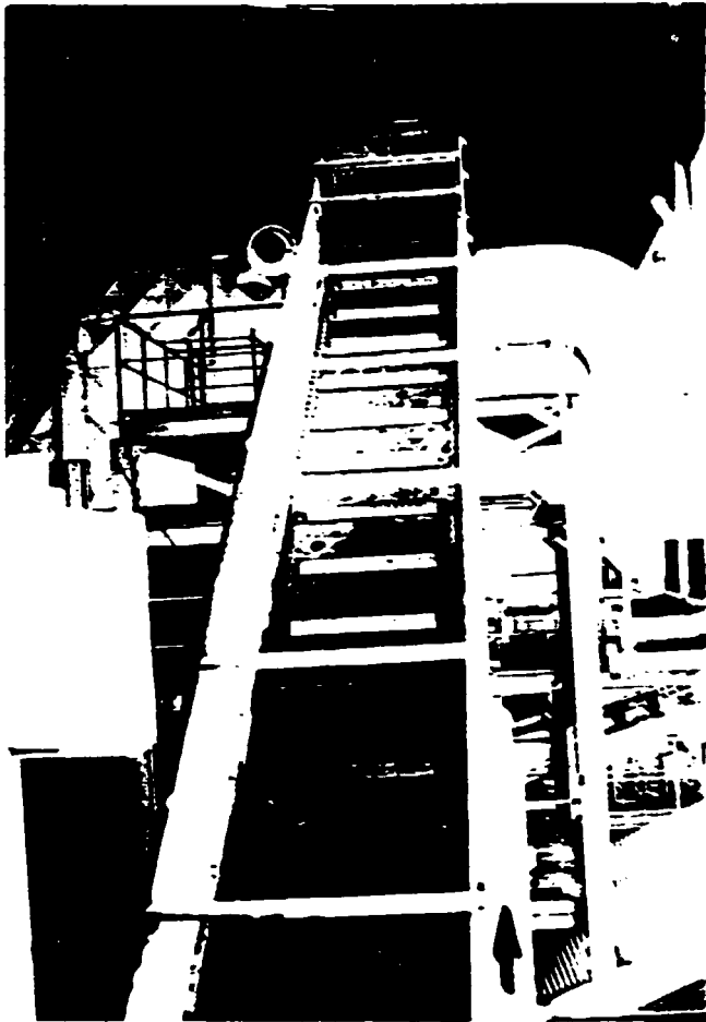
VIEW OF ASH CONVEYOR WITHOUT COVERING
