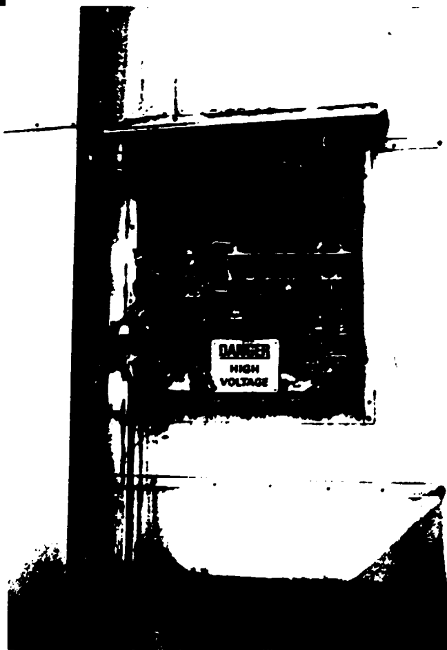
ELECTROSTATIC PRECIPITATOR VIEW OF EXTERNAL INSULATION DOOR OF HIGH VOLTAGE EQUIPMENT
