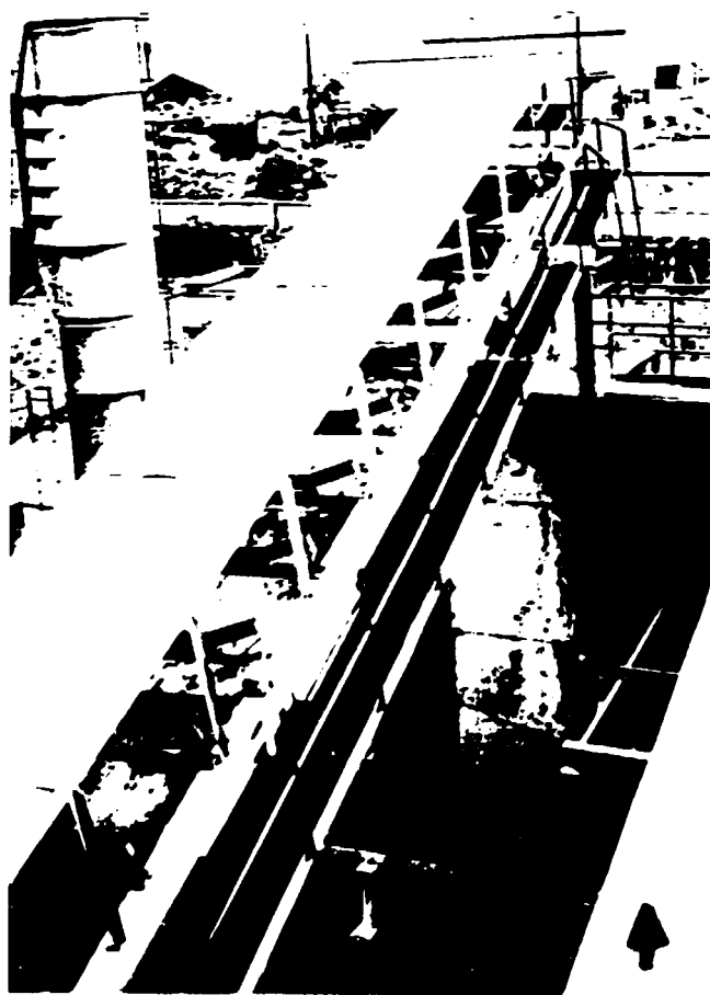
OUTLET ASH CONVEYER SYSTEM
