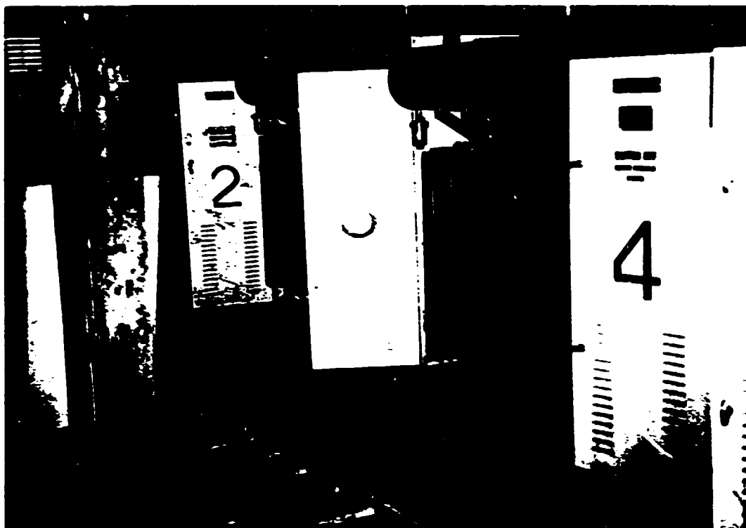
TRANSFORMER STATION (INTERIOR VIEW)
