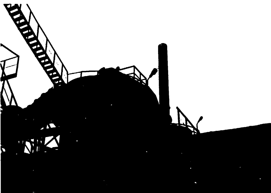
Short stack of absorption tower sulfuric acid plant
