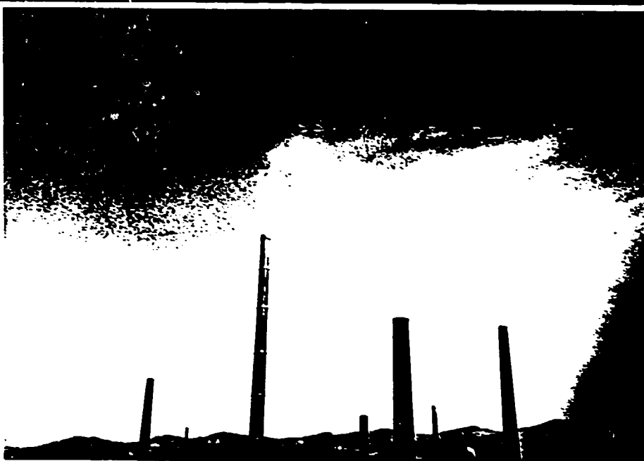
250 m stack in operation
