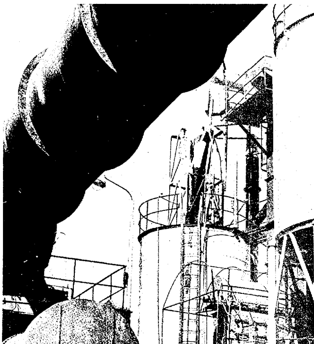
View of TCP Plant
