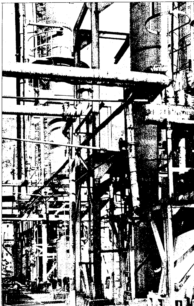
View of Formaldehyde Plant
