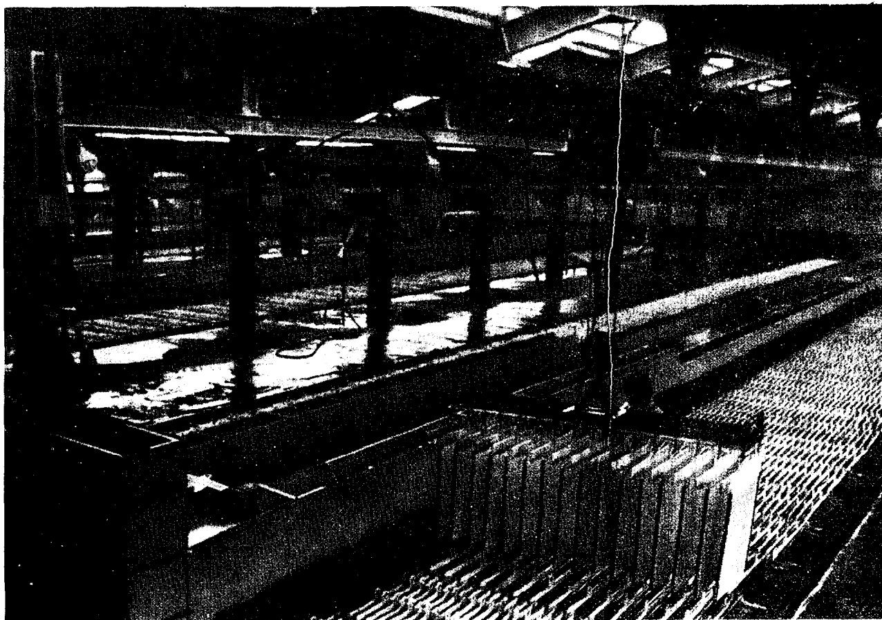
View of Zinc Electrolysis Facility
