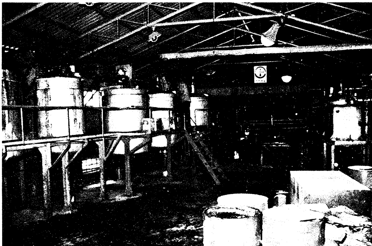
View of Mixing Equipment
