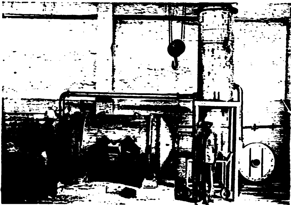
Electric Furnace for Melting and Refining Aluminum Alloy
