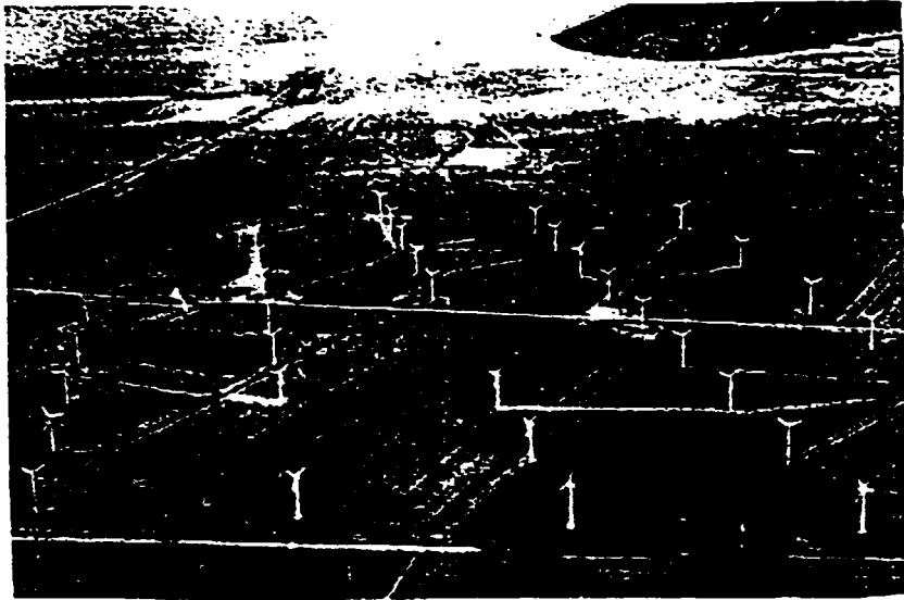
Aerial photo of a small windfarm
