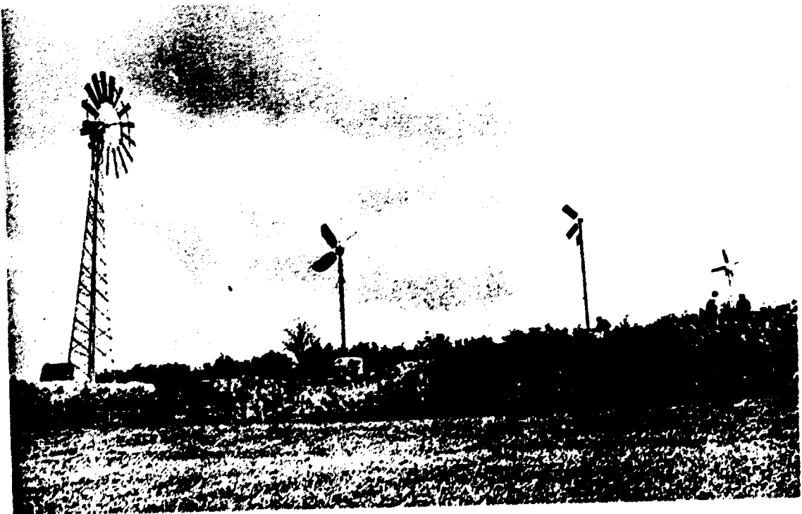
Small windpumps, electrical and mechanical, at the Test Station
