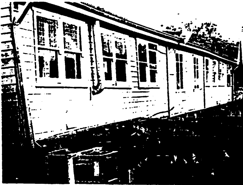
(building has been moved sideways off footings)
