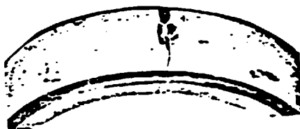
Fig. 26 Outer ring shell surface of a grooved ball bearing 6309 with the impression of a pressure screw and a transversal crack.
