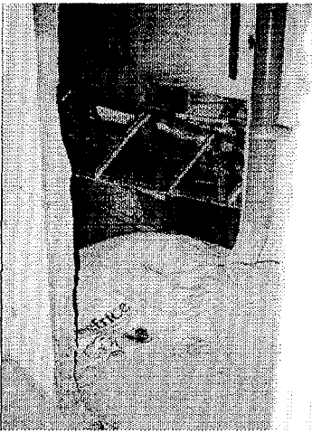
Heavy residue build up
