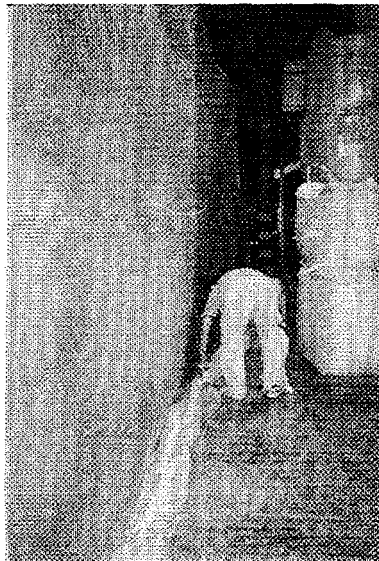
Use sand snakes to seal stacks
