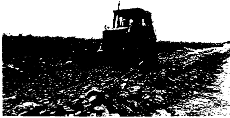
Photo 5: Preparation of landfill site / dike
