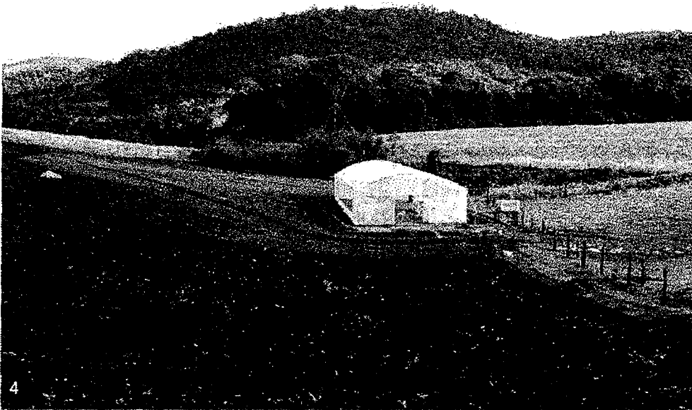
Figure 6. High metallic tunnel, Ituporanga, Santa Catarina
