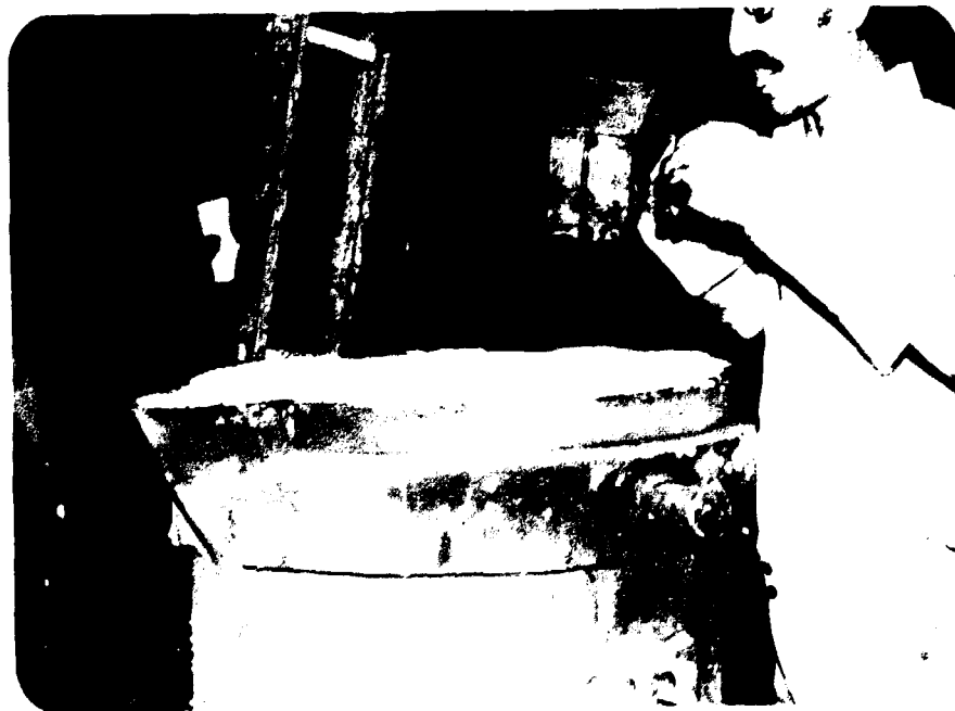
Fig. 62 KEEPING THE MAGNESIUM ALLOY IN THE POCKET OF THE SPECIAL LADLE
