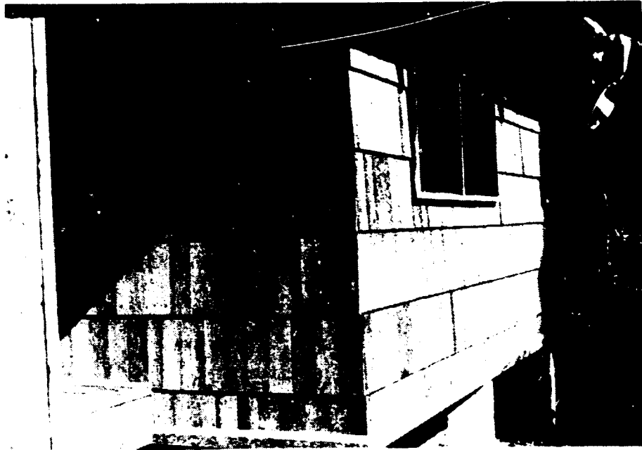
Detail of wall shingle application.
