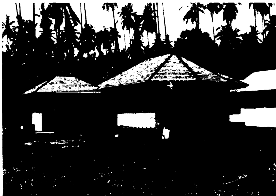
"Tongian" design with modified hip type of roof - concrete slab flooring and masonry walls up to 1.75 metres from floor level.
