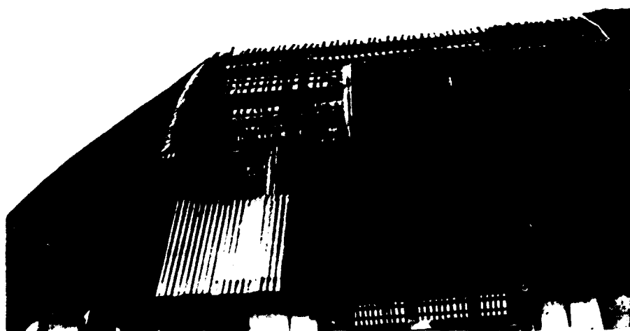
Similar church building at the FOA island (Ha'apai group of Tonga Islands) partly damaged by Hurricane "Issac" (blow out roofing sheets) - roof structural C.P.W. slightly damaged. Age of church approximately 60-80 years. See horizontal nailing battens added to roof when thatching was replaced by metal sheet cover.
