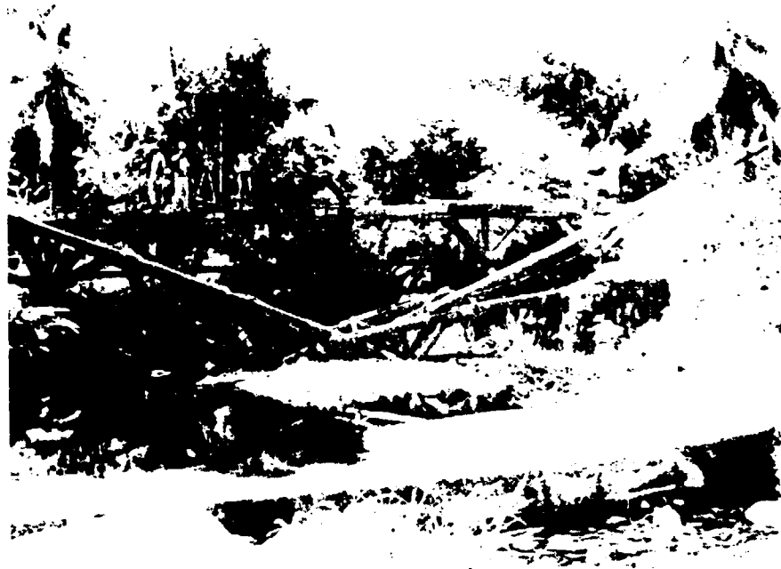
Fig. 12 Collapsed Girder
