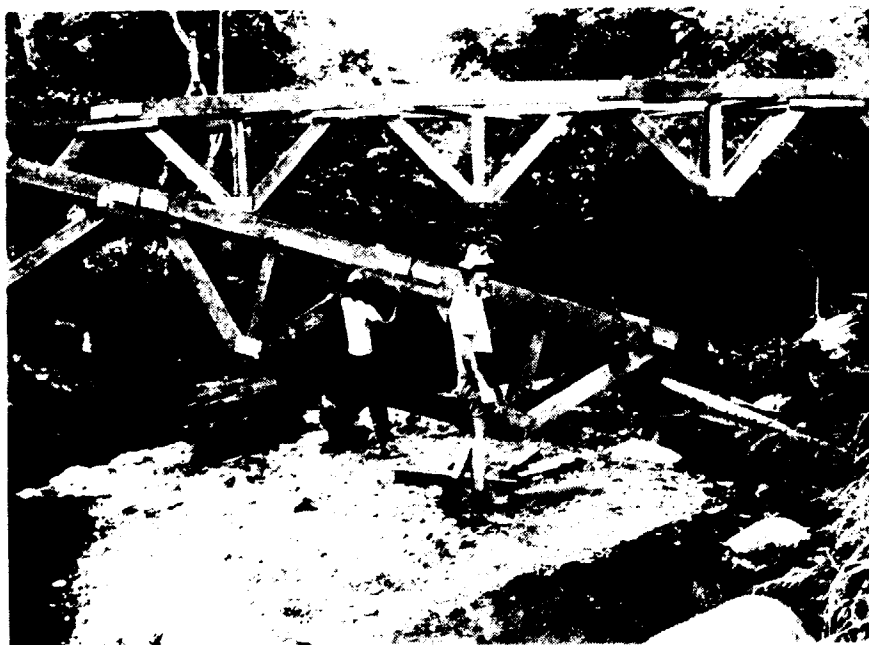
Fig 15 Girder Being raised
