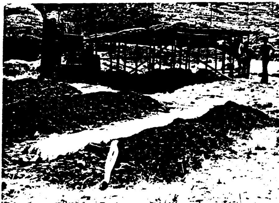
Fig. 12 Debre Zeyit (ILCA) In the background: roofed-in plastic plug flow digester, length 7 m In the foreground: small polythene plug flow diges ter in shallow trench.
