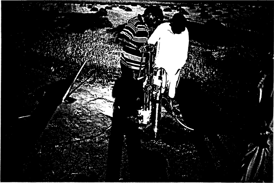
Photograph 3 Concrete Sampling with Drill Press Mounted Core Cutting Machine
