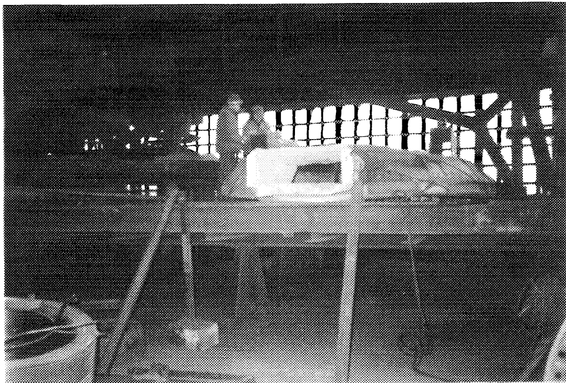
Plate 6: Scan Lance Roof During Maintenance - Showing Rear Extraction Port
