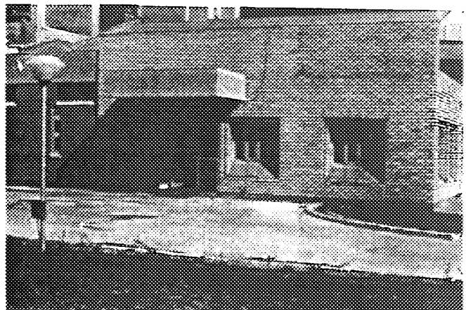
House constructed with Sand Lime Flyash Bricks
