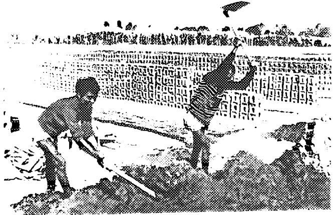
Manual mixing of raw materials for production of Clay-Flyash Bricks
