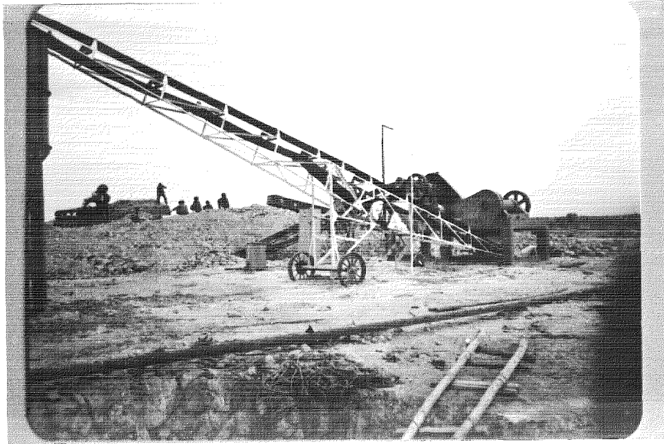
Fig. 1 Two-stage open-circuit crushing unit
