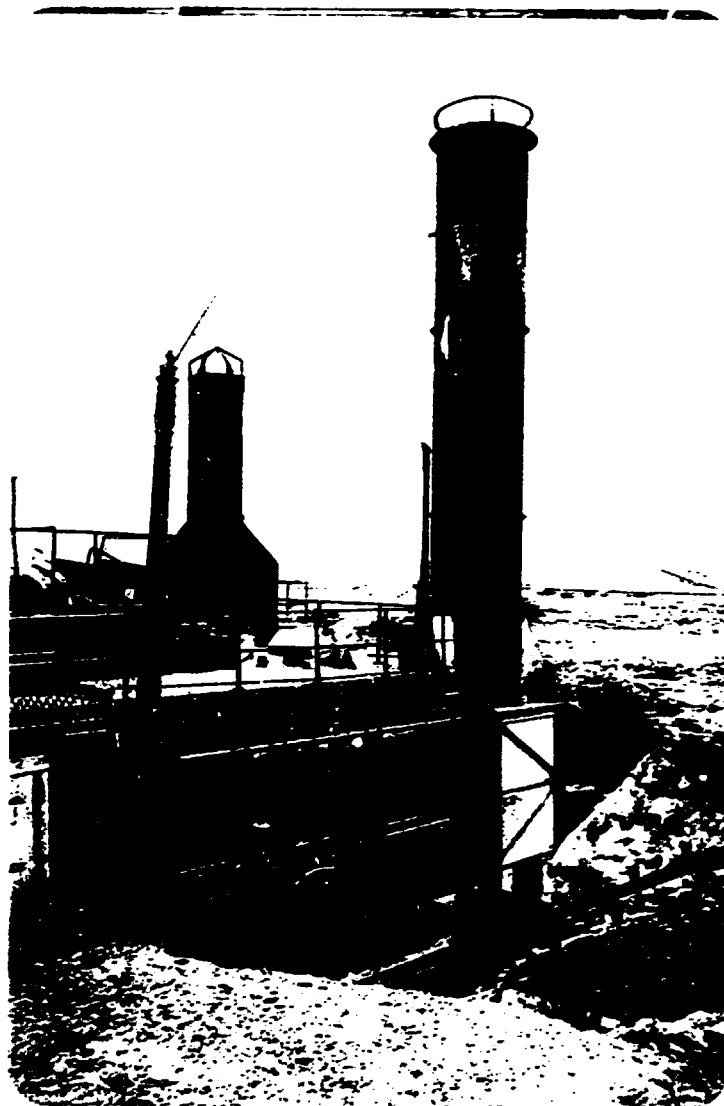
Medical waste incinerator at Awali
