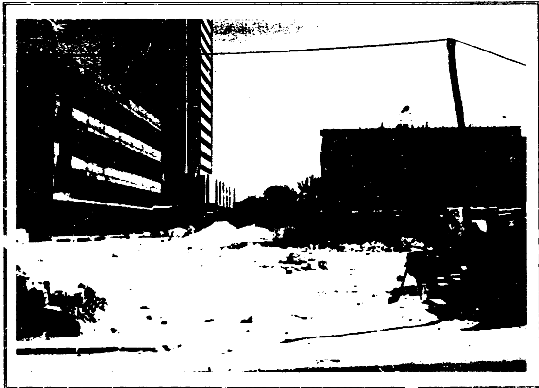
BUILDINGS UNDER CONSTRUCTIONS
