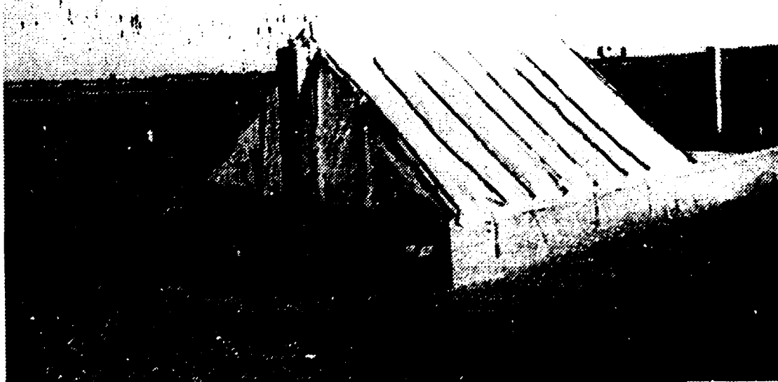
PHOTOGRAPH 6 TEMPORARY SOLAR STILL - 4050 MM X 3600 MM
