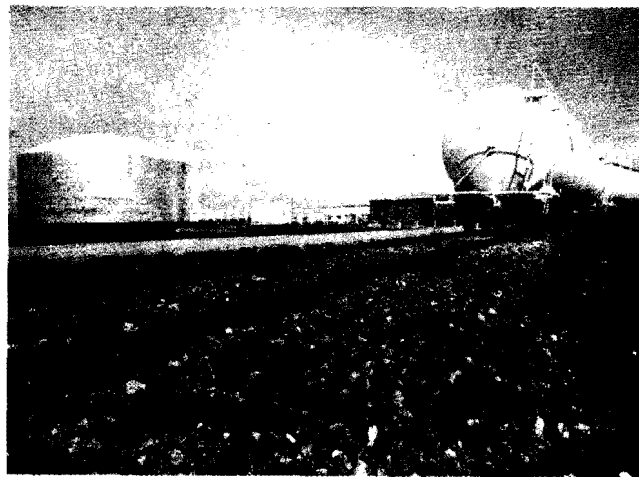
Figure 8. Large Storage Terminal that Receives Ammonia by Rail.
