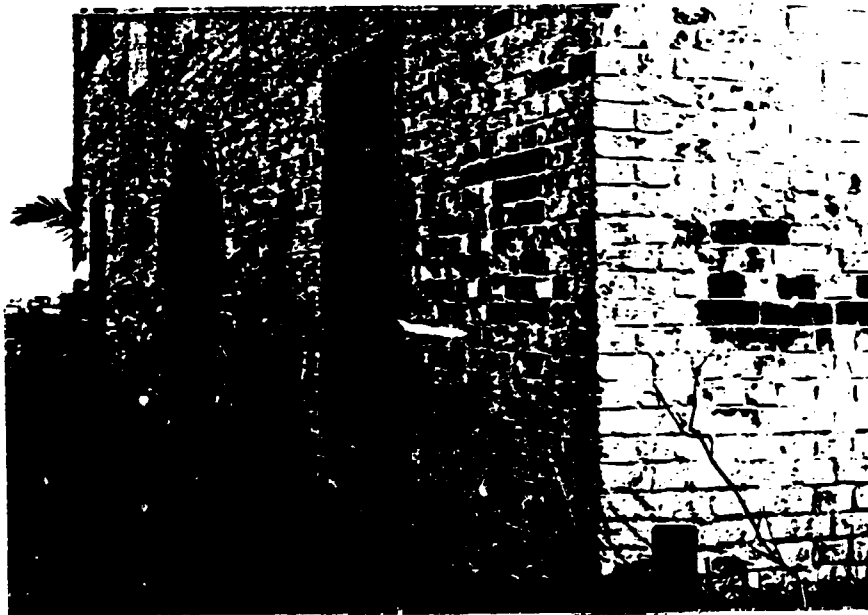
A corner of the Legislature Building in Koror. Showing the fired clay brick work beneath a surface decorative coating.
