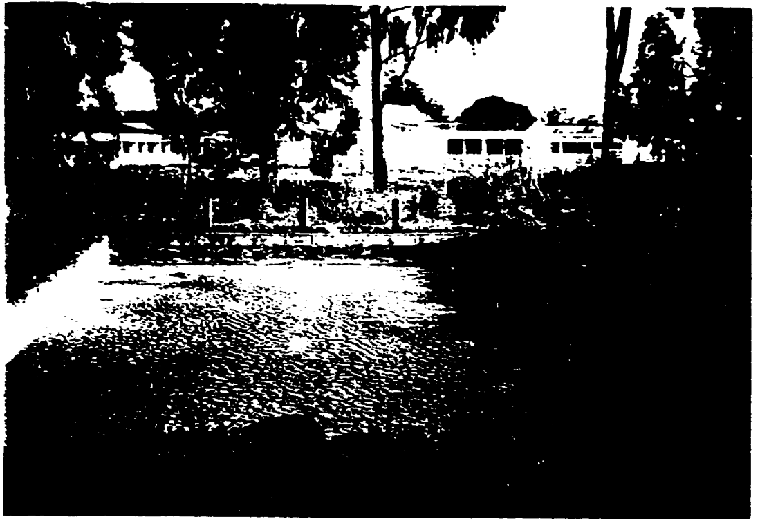
Photo 9. Chrome sludge is dried in chrome sludge beds before final disposal.
