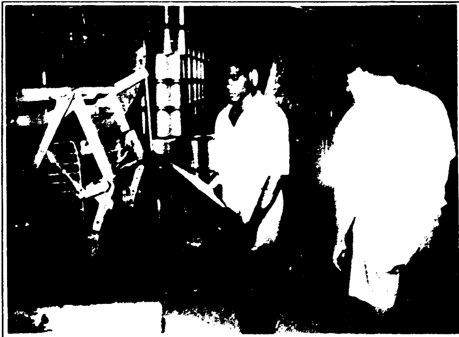
Figure 4. A worker being supervised by the workshop owner in retrieving a piece of oil drum cover from a stamping machine.
