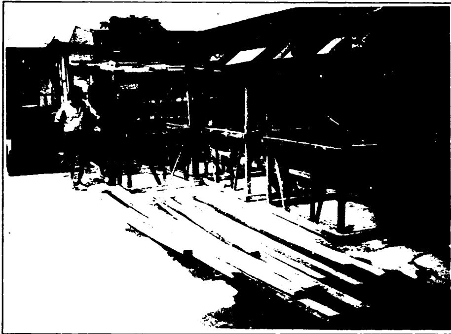
Figure 3. Some of the chilli drier wood frames fabricated by a joinery and ready for fitting with metal pipes which will serve as heat exchangers between the furnace and the heating chamber of the drier.
