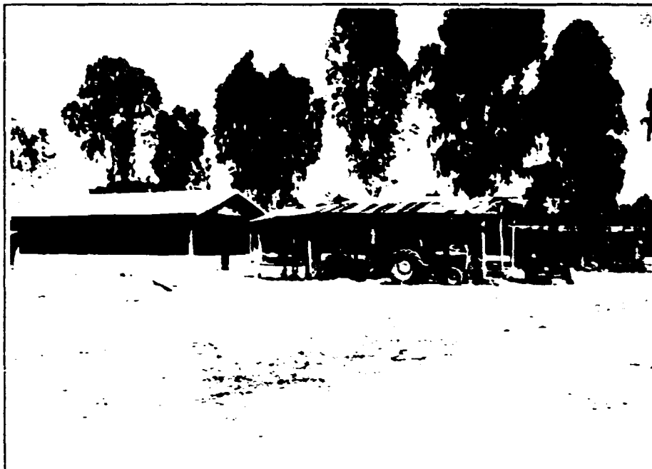
Figure 11. The Nabong Agricultural College tractor and machinery sheds and workshop.
