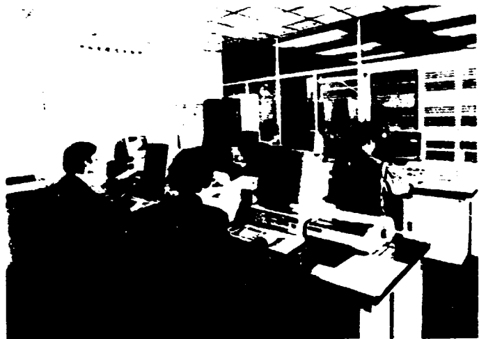
The control room at Yingkou's telecommunications centre.
