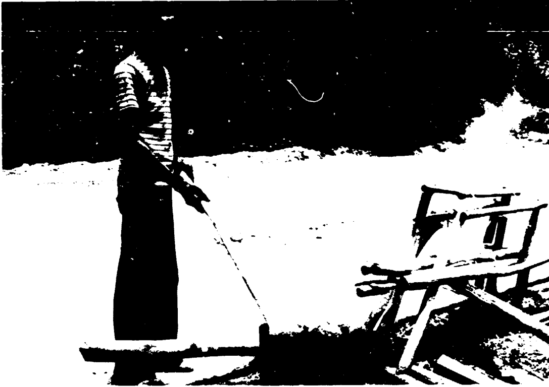
Conventional Drum Charcoaling in the Field
