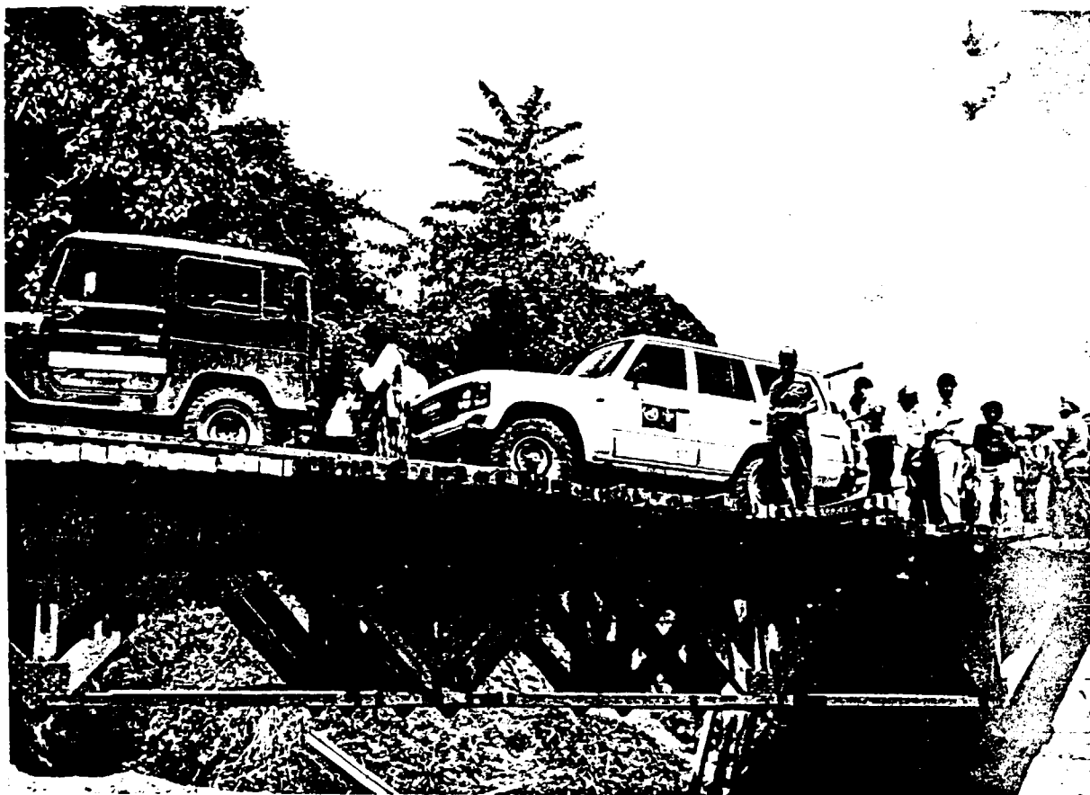
Figure 3. Partially completed bridge during launching ceremony.
